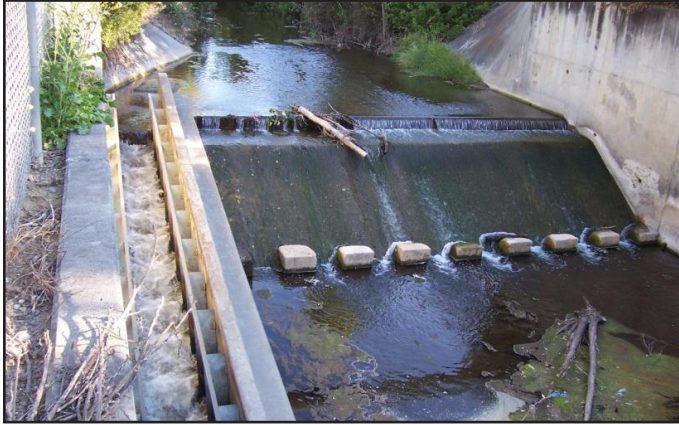
Example of a fish ladder to be modified or reconstructed for improved fish passage
