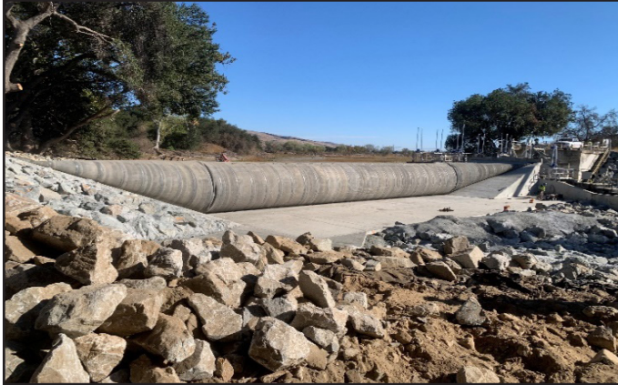
Phase 1 of the Coyote Percolation Dam has been completed, and the image shows the newly installed inflated bladder dam
